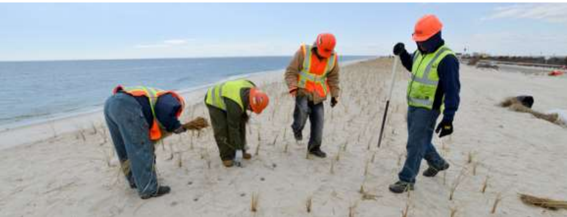
Hither Hills State Park – post-Hurricane Sandy restoration work
