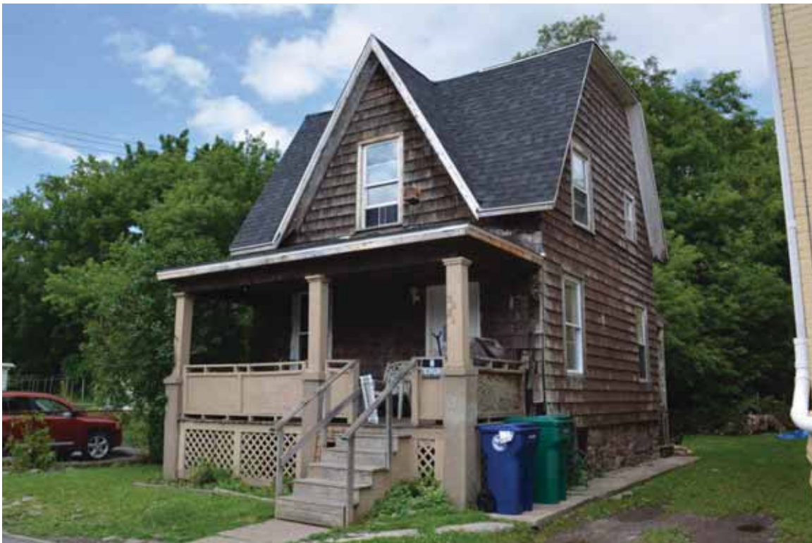
Photograph 4.144. 2655 Spring Street, facing northeast (Panamerican 2014).
