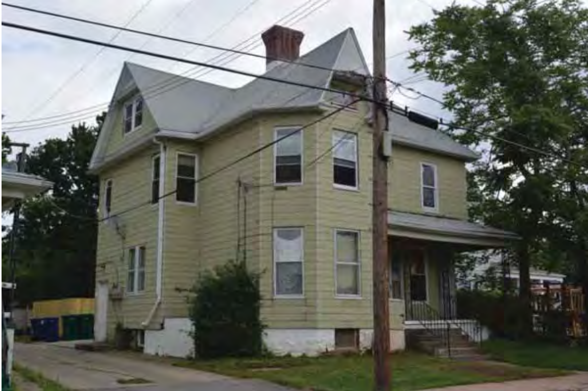
Photograph 4.109. 726 Linwood Avenue, facing northeast (Panamerican 2014).
