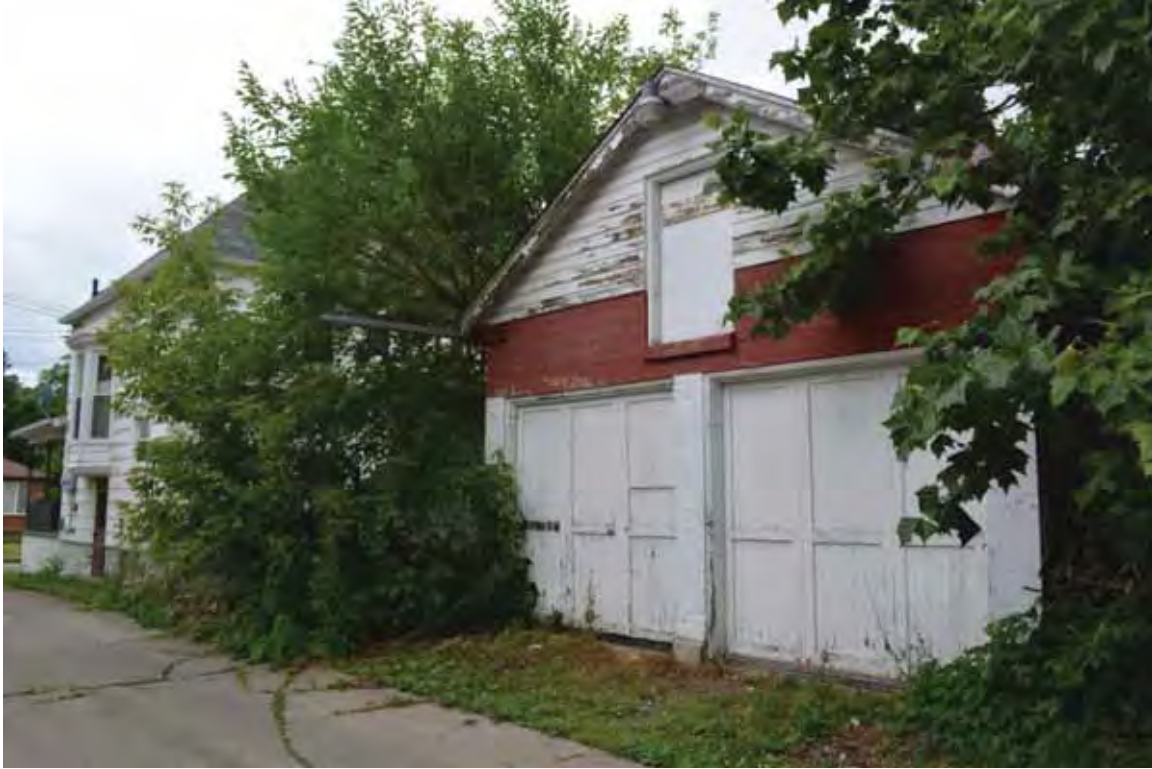
Photograph 4.107. 716A Linwood Avenue, facing southwest (Panamerican 2014).
