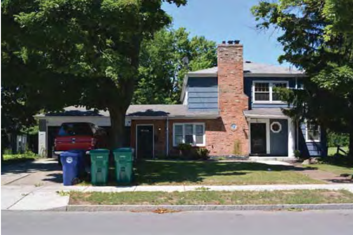
Photograph 4.99. 2848 Lewiston Road, facing west (Panamerican 2014).
