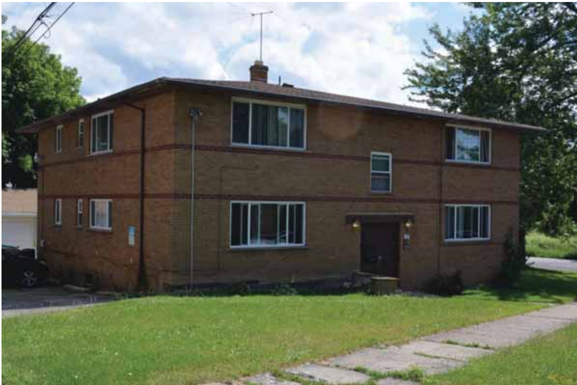
Photograph 4.56. 605 Chasm Avenue, facing southeast ( Panamerican 2014 ).
