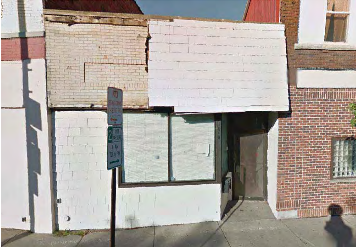
Photograph 4.120. 1410 Main Street, facing west (Google Earth 2015).
