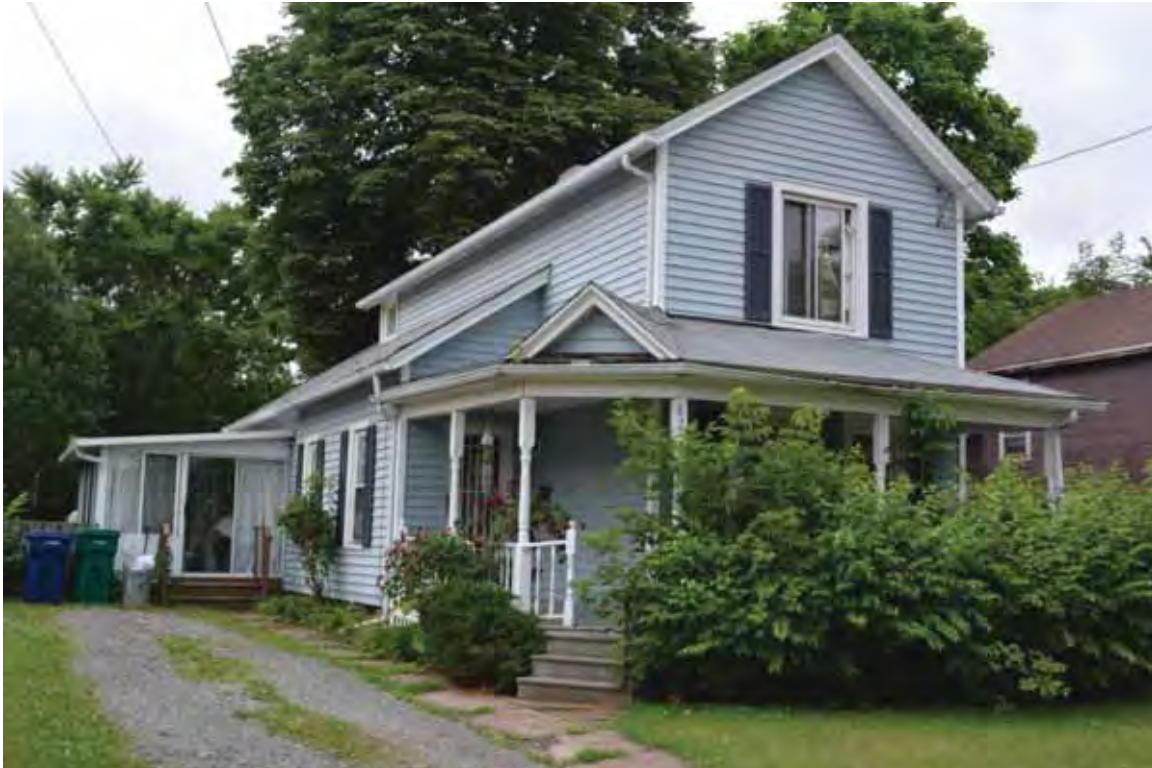
Photograph 4.198. 825 Willow Street, facing southwest (Panamerican 2014).
