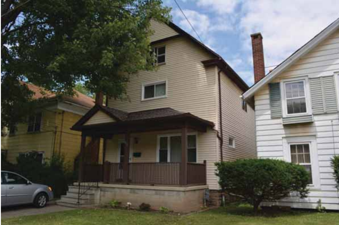
Photograph 4.101. 818 Lincoln Place, facing northwest ( Panamerican 2014 ).
