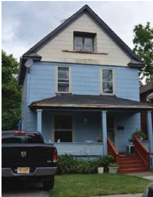
Photograph 4.192. 810 Willow Street, facing north (Panamerican 2014).
