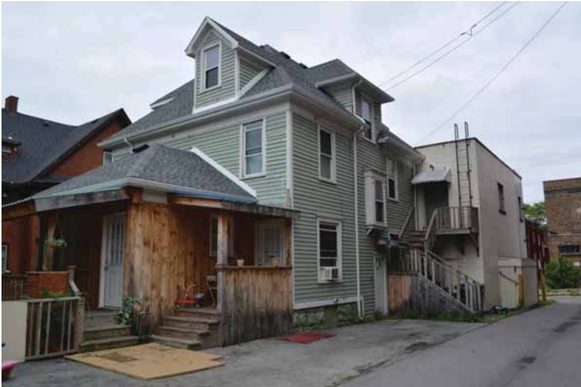
Photograph 4.74. 811 Division Avenue, facing northwest (Panamerican 2014).
