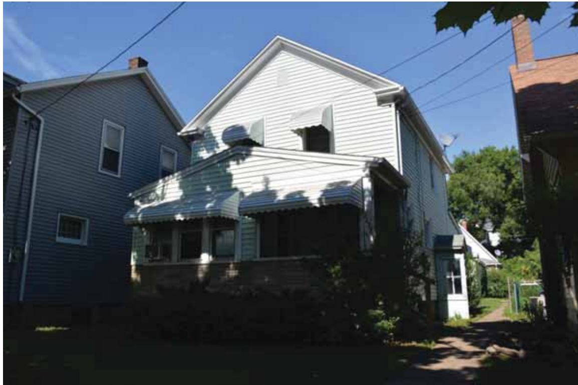
Photograph 4.170. 2673 Whirlpool Street, facing east (Panamerican 2014).
