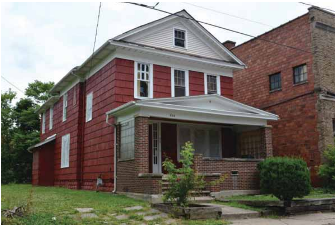
Photograph 4.75. 814 Division Avenue, facing northeast (Panamerican 2014).
