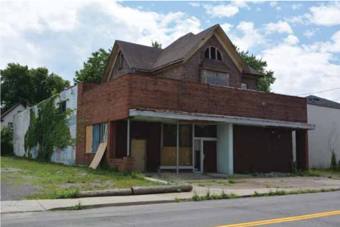
Photograph 4.68. 813 Cleveland Avenue, facing southwest (Panamerican 2014).
