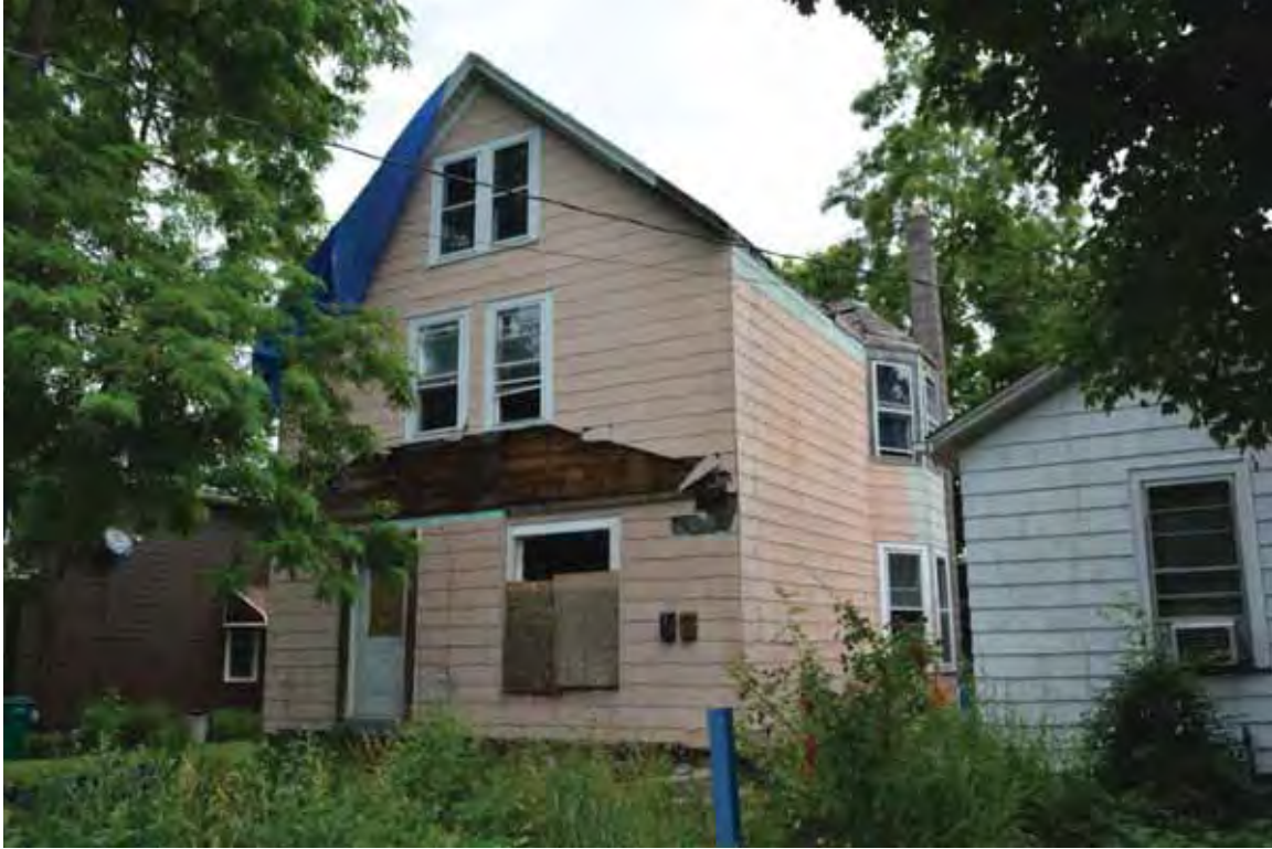
Photograph 4.85. 1509 Eighth Street (vacant), facing northeast (Panamerican 2014).
