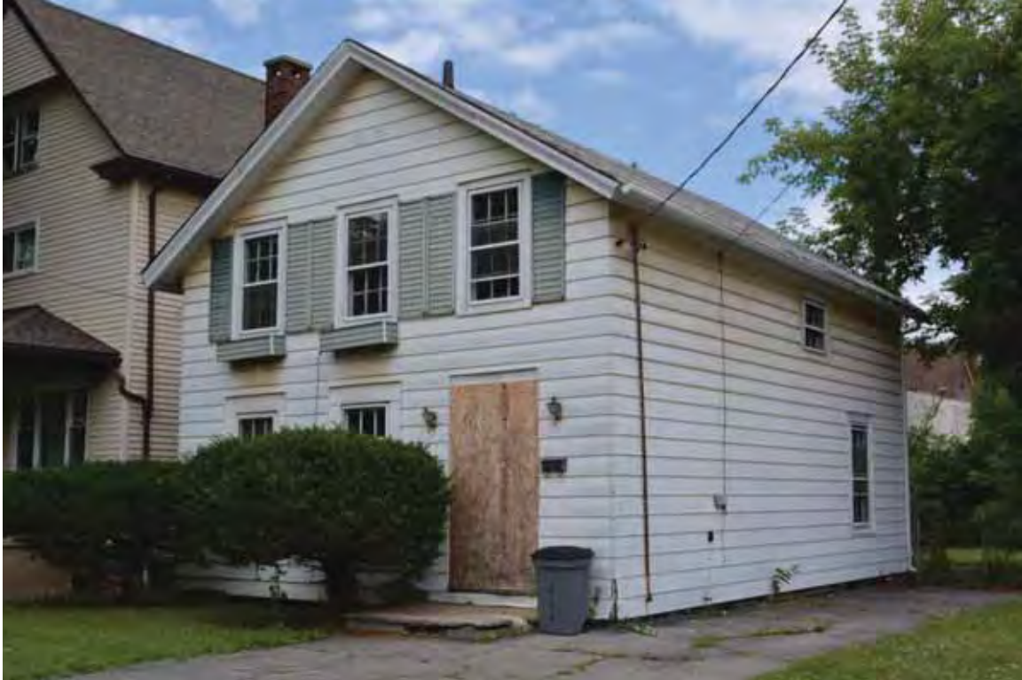
Photograph 4.103. 824 Lincoln Place, facing northwest (Panamerican 2014).
