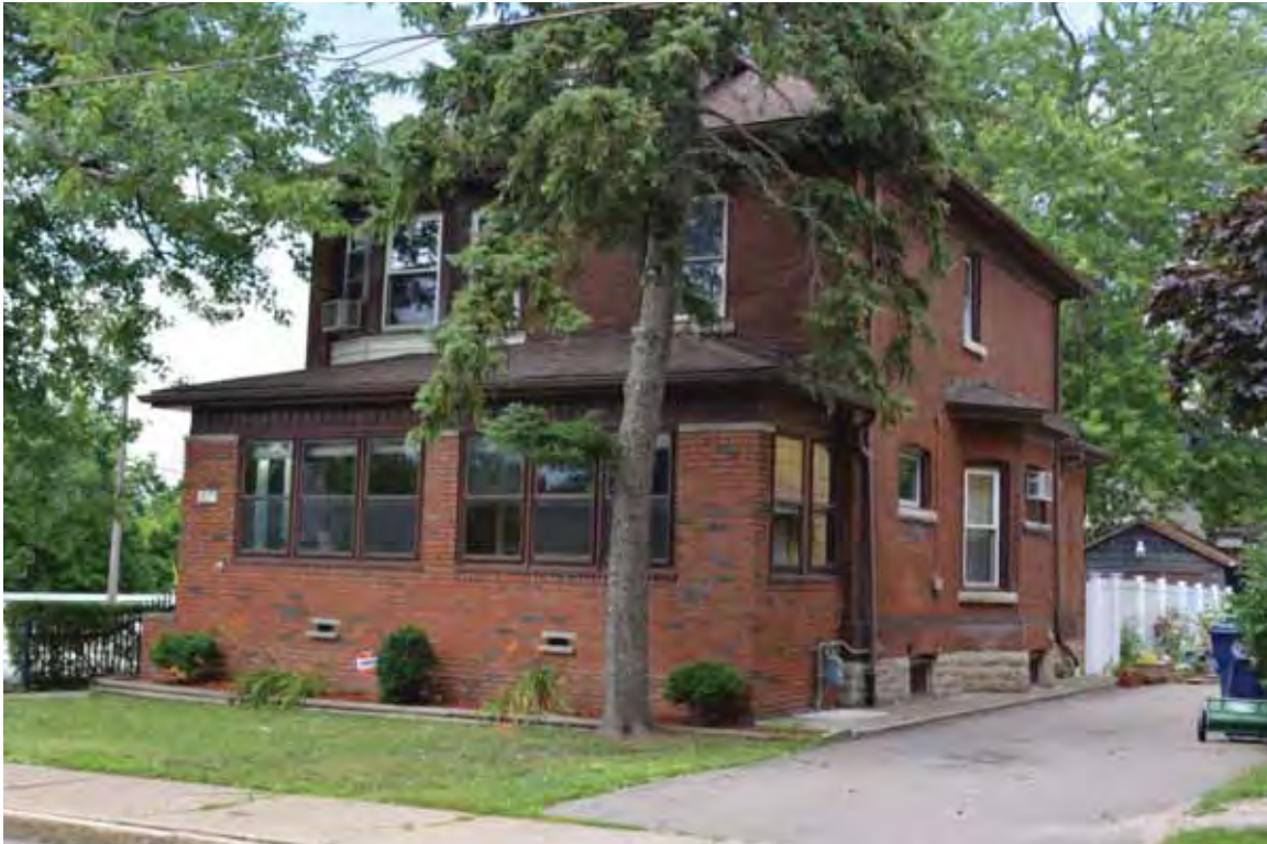
Photograph 4.100. 812 Lincoln Place, facing northwest (Panamerican 2014).
