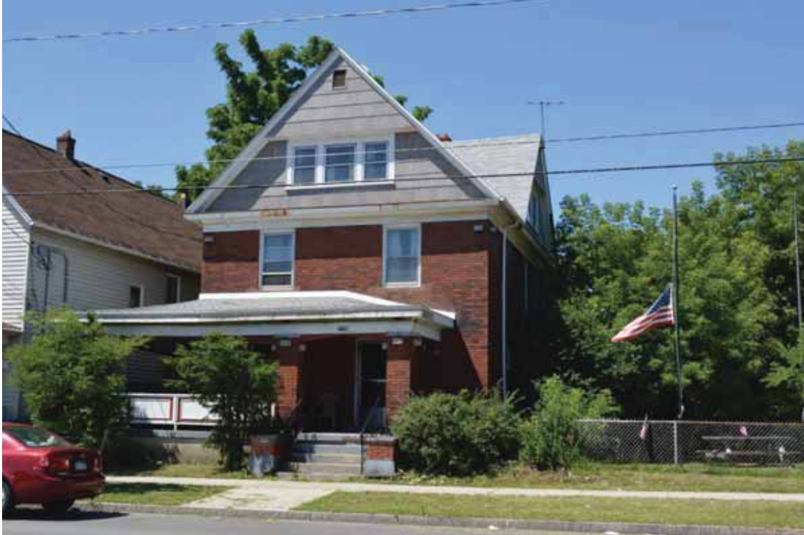
Photograph 4.139. 2726 Main Street, facing west-southwest (Panamerican 2014).
