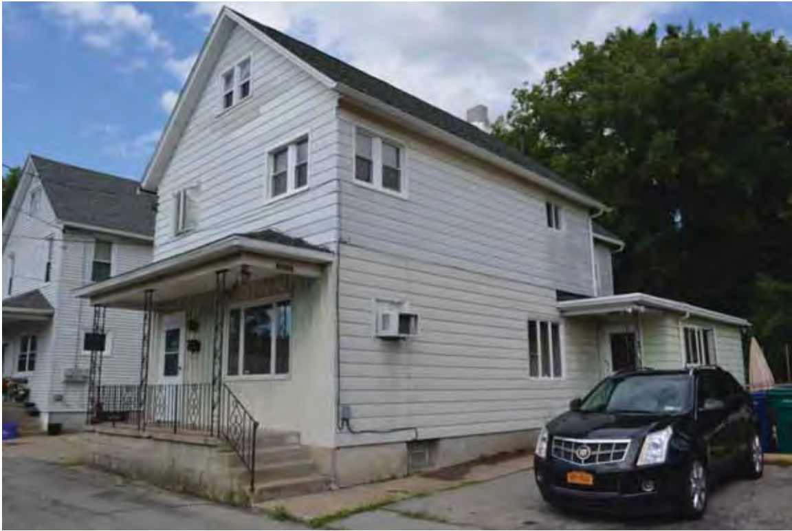
Photograph 4.145. 2657 Spring Street, facing northeast (Panamerican 2014).
