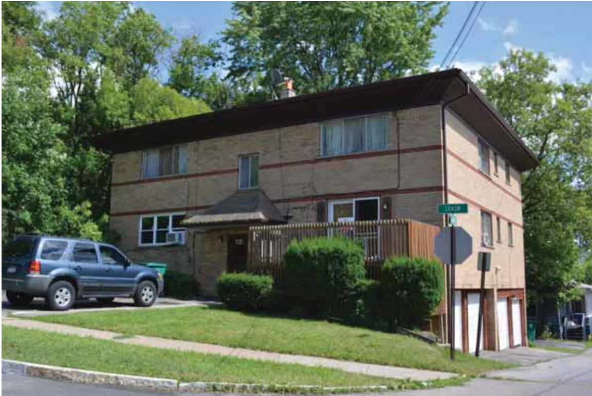
Photograph 4.58. 611 Chasm Avenue, facing southeast (Panamerican 2014).
