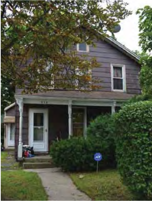
Photograph 4.195. 819 Willow Street, facing south (Panamerican 2014).
