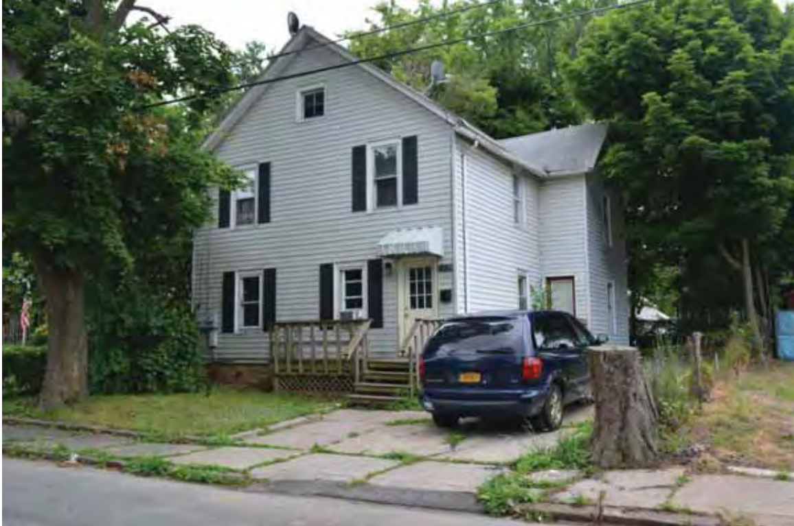
Photograph 4.187. 721 Willow Street, facing southeast (Panamerican 2014).
