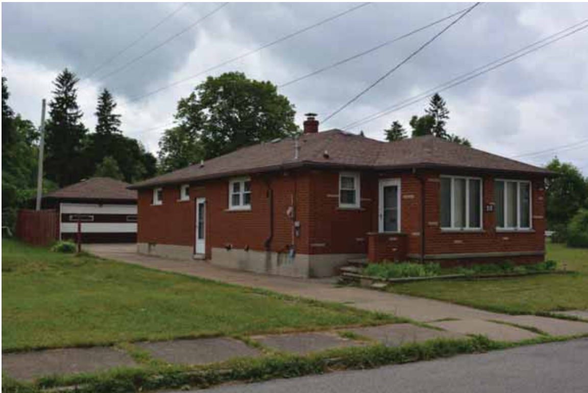
Photograph 4.108. 717 Linwood Avenue, facing southwest (Panamerican 2014).
