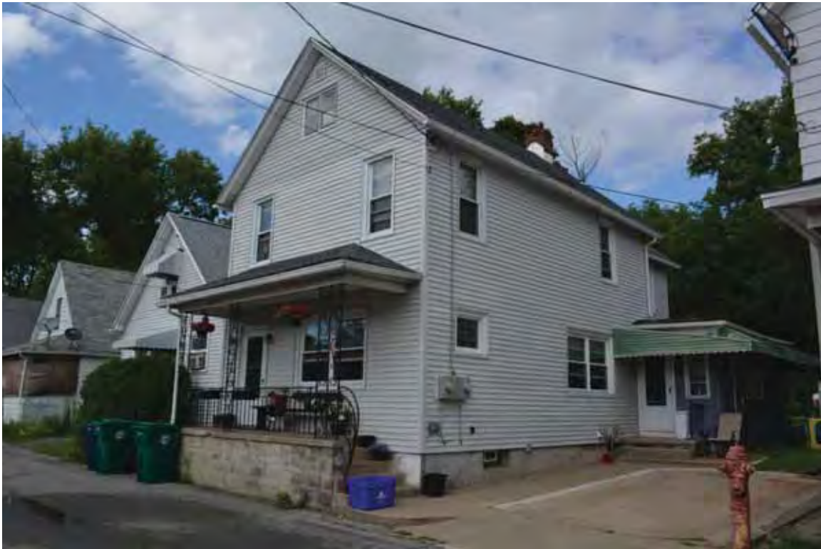
Photograph 4.146. 2659 Spring Street, facing northeast (Panamerican 2014).
