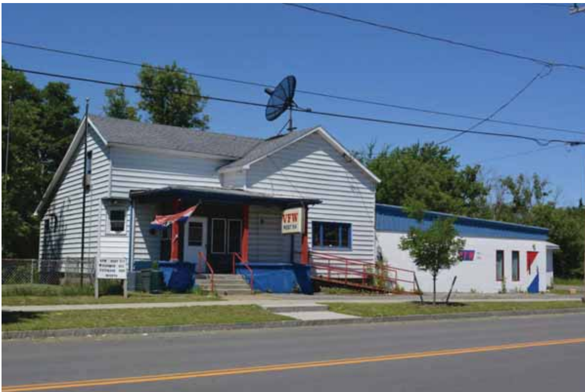
Photograph 4.140. 2772 Main Street, facing northwest (Panamerican 2014).
