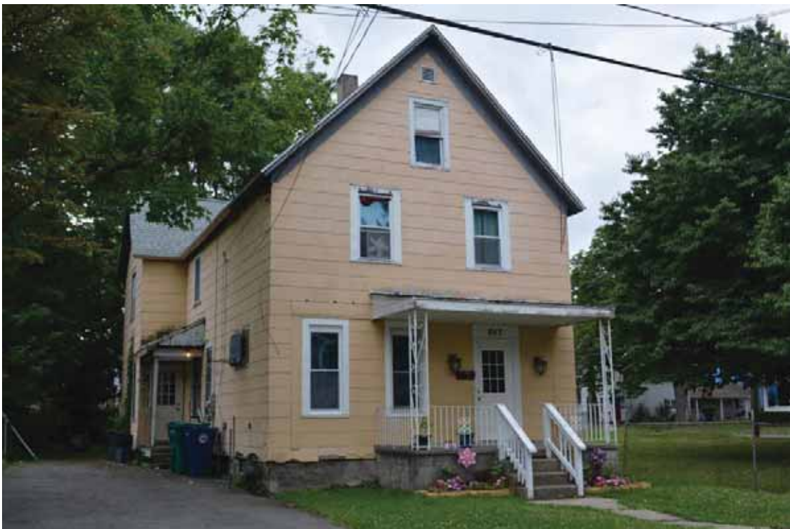
Photograph 4.190. 807 Willow Street, facing south (Panamerican 2014).
