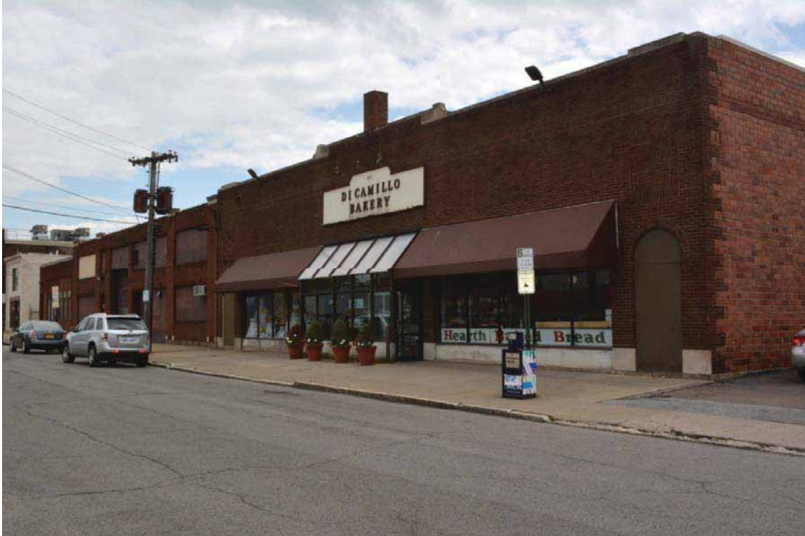
Photograph 4.111. 801 Linwood Avenue, facing southeast (Panamerican 2014).
