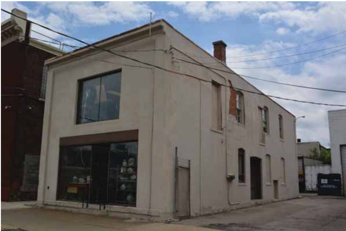
Photograph 4.114. 831 Linwood Avenue, facing southeast (Panamerican 2014).
