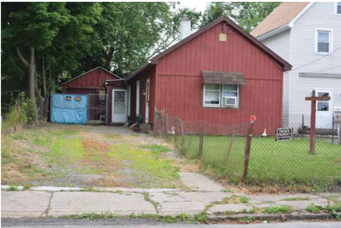
Photograph 4.186. 717 Willow Street, facing south (Panamerican 2014).
