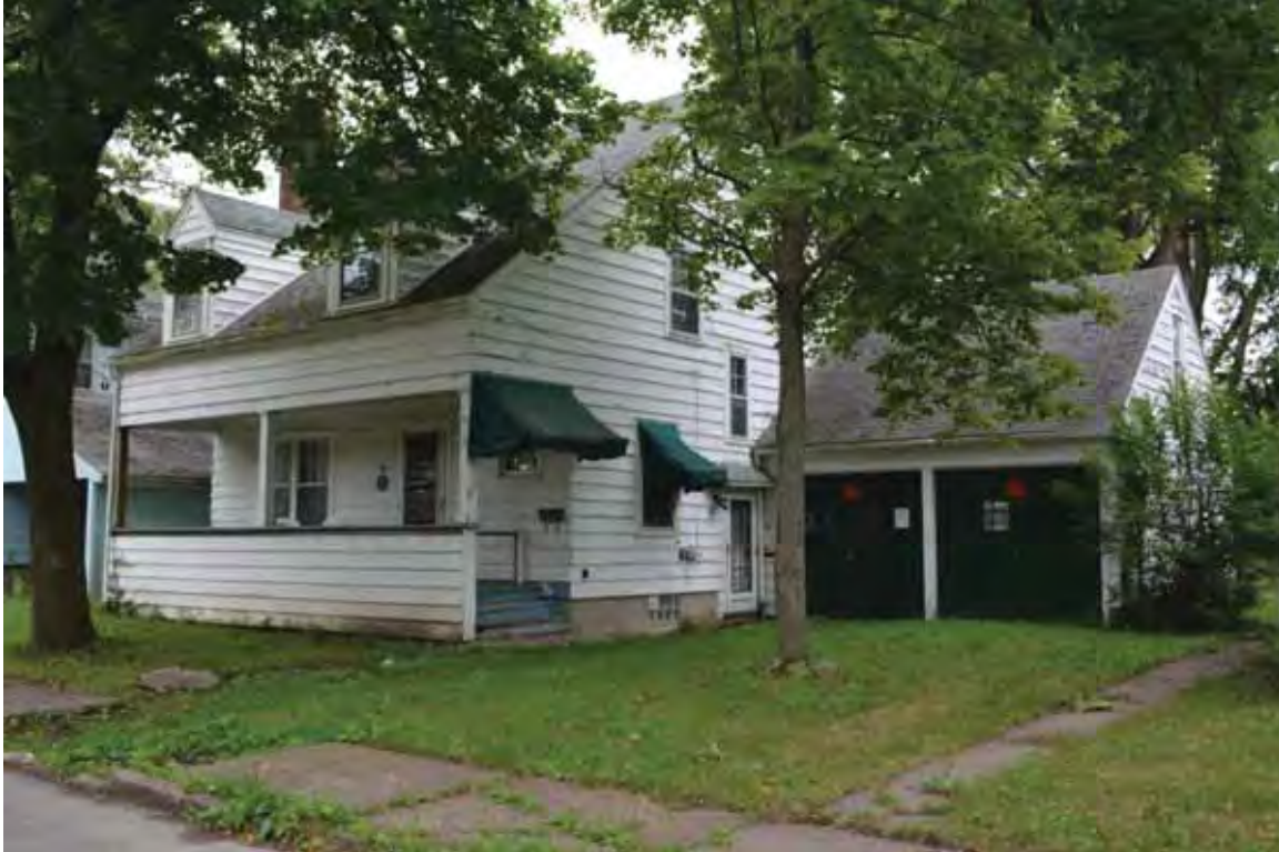
Photograph 4.189. 735 Willow Street, facing southeast (Panamerican 2014).
