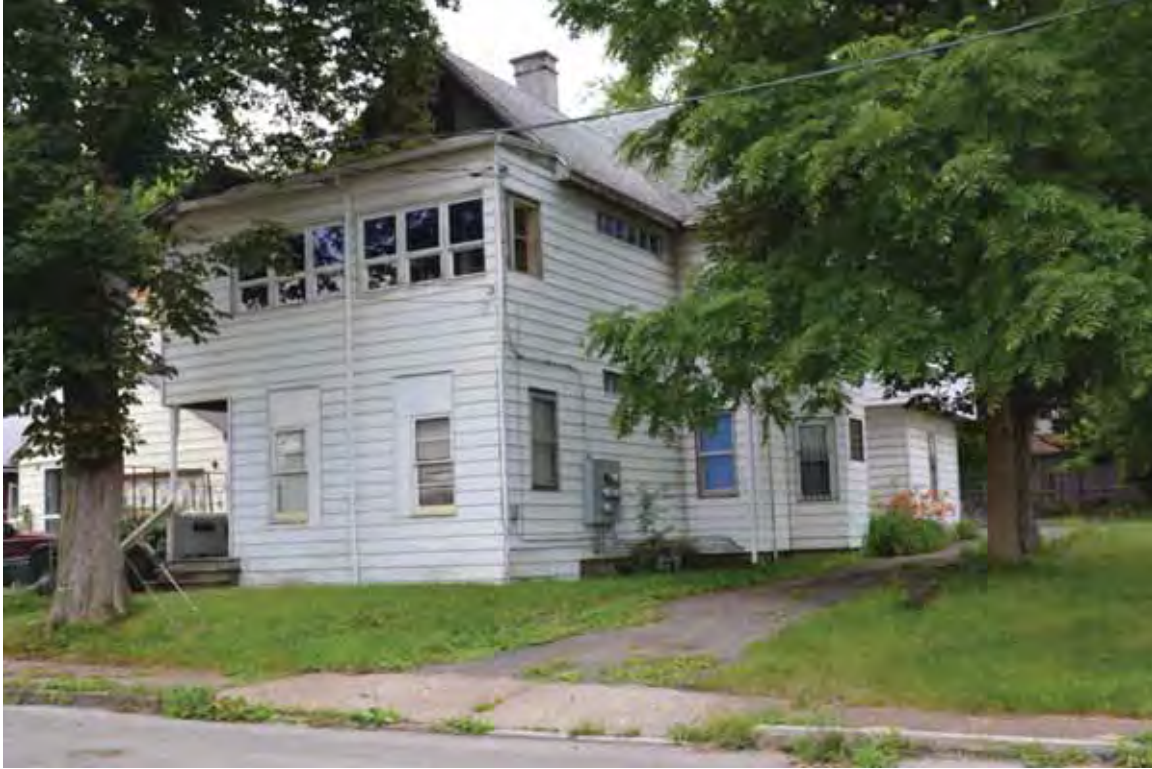
Photograph 4.183. 711 Willow Street, facing southeast (Panamerican 2014).
