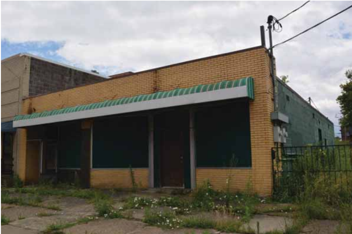
Photograph 4.104. 833 Lincoln Place, facing southeast (Panamerican 2014).
