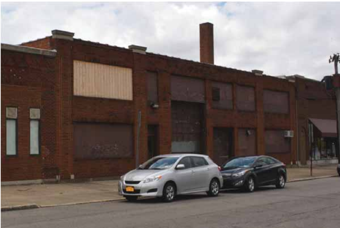
Photograph 4.112. 827 Linwood Avenue, facing southwest (Panamerican 2014).
