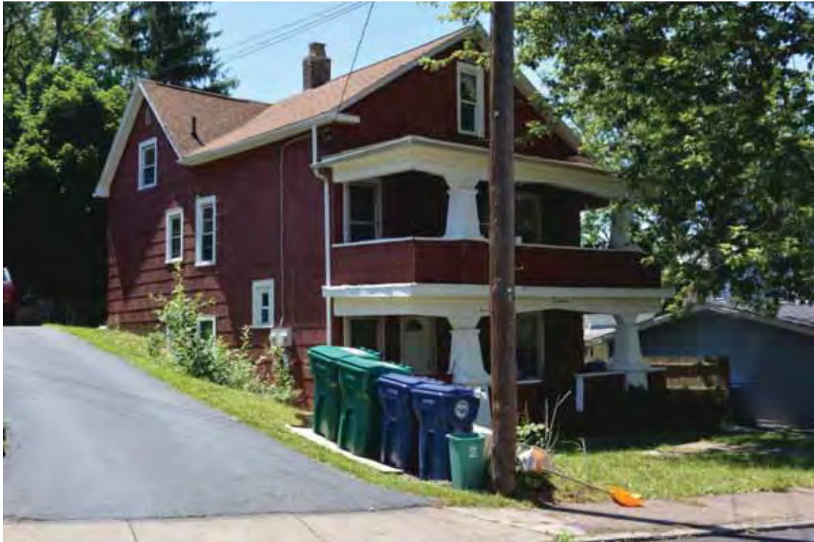
Photograph 4.61. 613 Chestnut Avenue, facing southwest ( Panamerican 2014 ).
