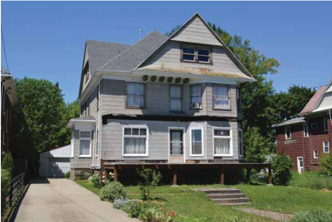
Photograph 4.94. 2808 Lewiston Road, facing west (Panamerican 2014).
