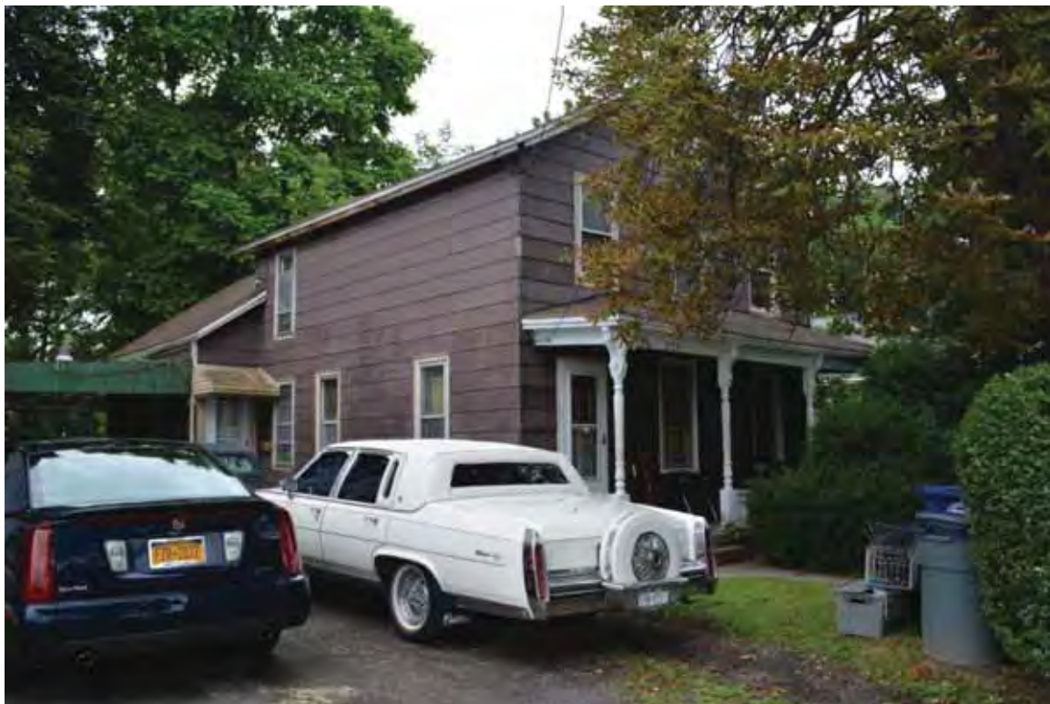
Photograph 4.196. 819 Willow Street, facing southwest (Panamerican 2014).
