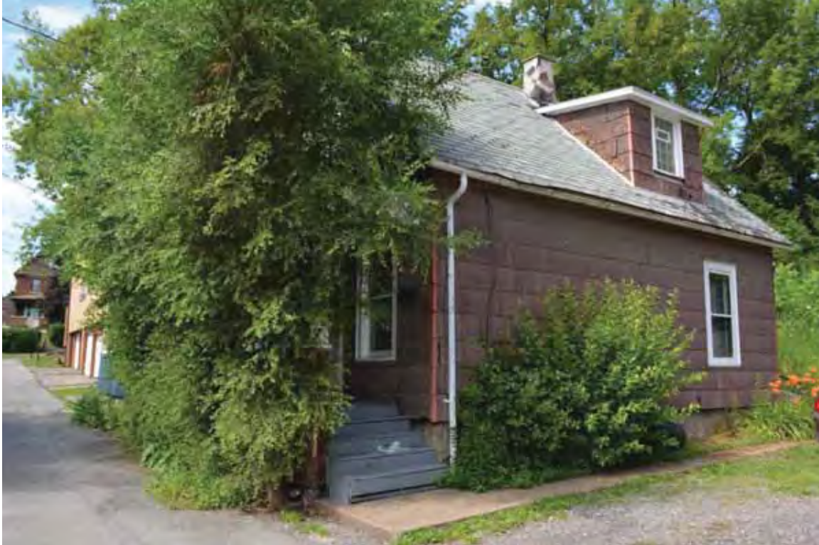
Photograph 4.151. 2679 Spring Street, facing northeast (Panamerican 2014).
