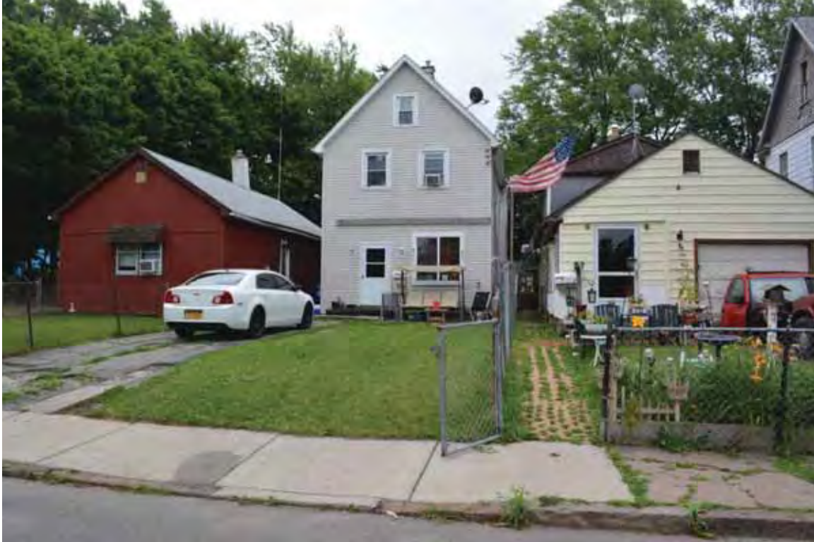
Photograph 4.185. 715 Willow Street, facing south (Panamerican 2014).
