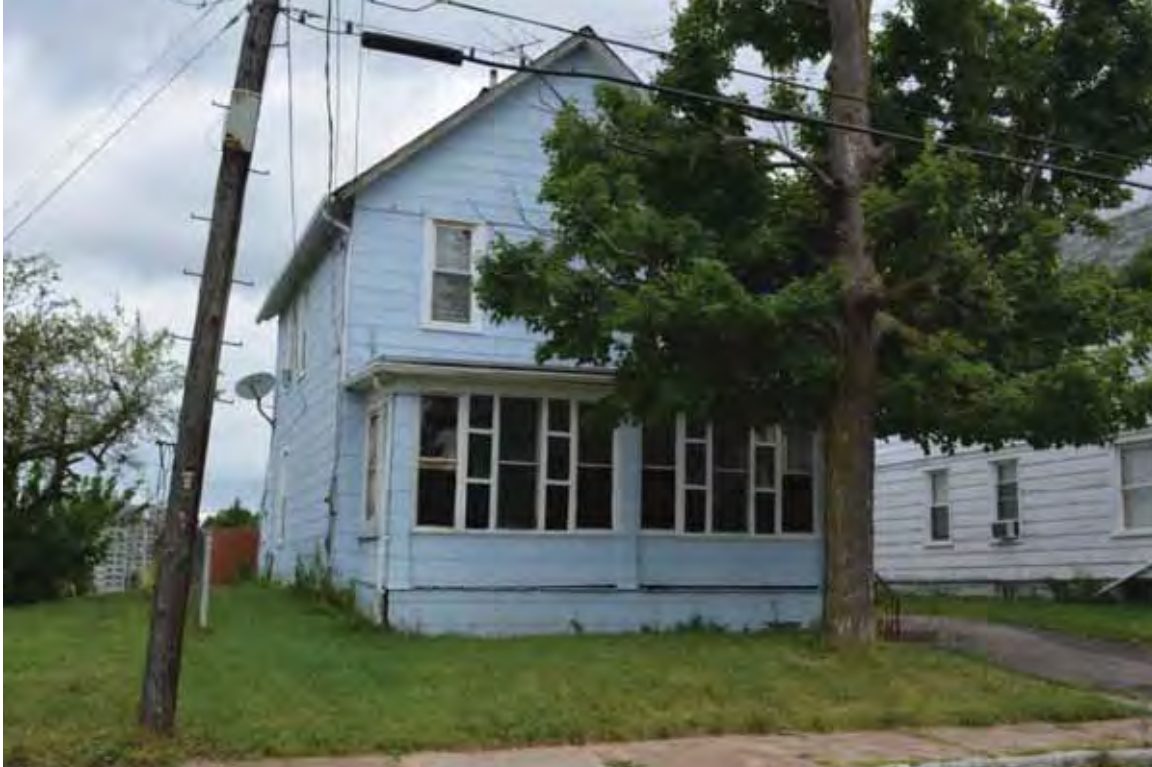
Photograph 4.105. 714 Linwood Avenue, facing north (Panamerican 2014).
