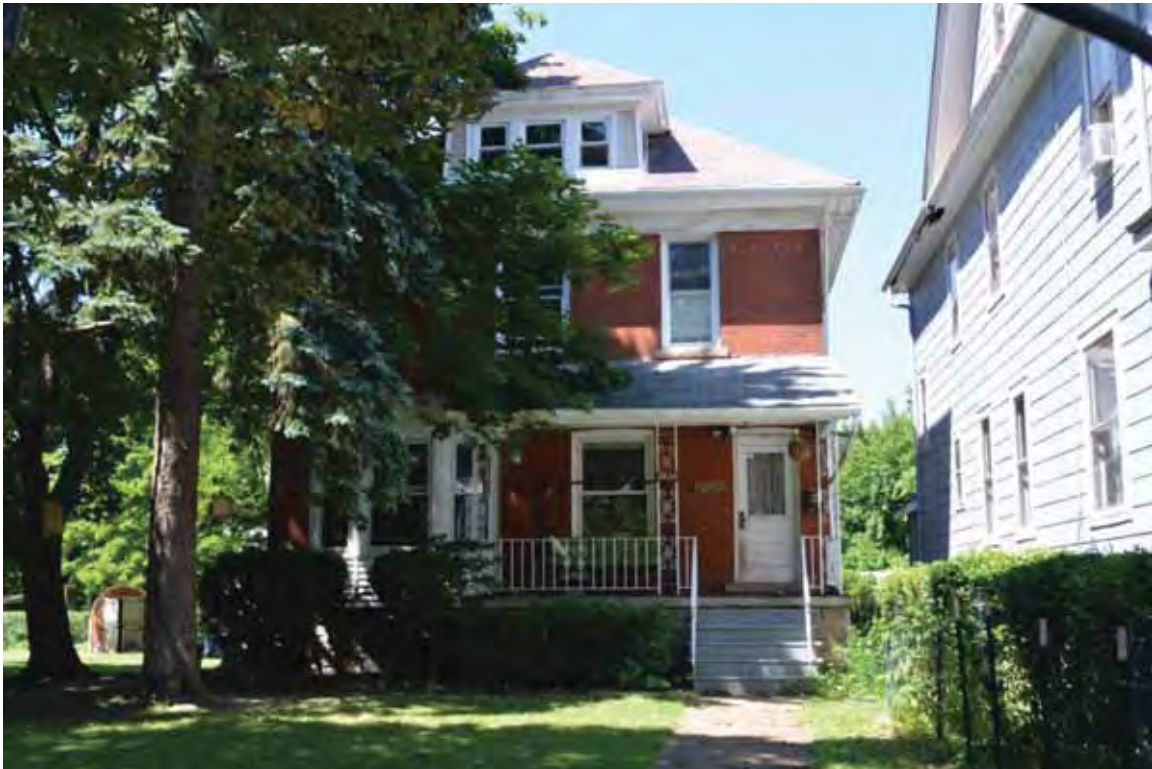
Photograph 4.96. 2834 Lewiston Road, facing west ( Panamerican 2014 ).
