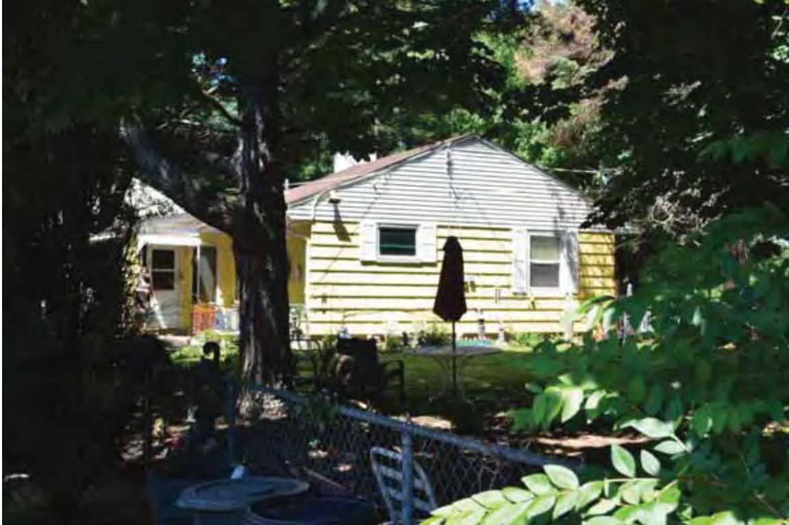
Photograph 4.65. 622½ Chestnut Avenue, facing west ( Panamerican 2014 ).
