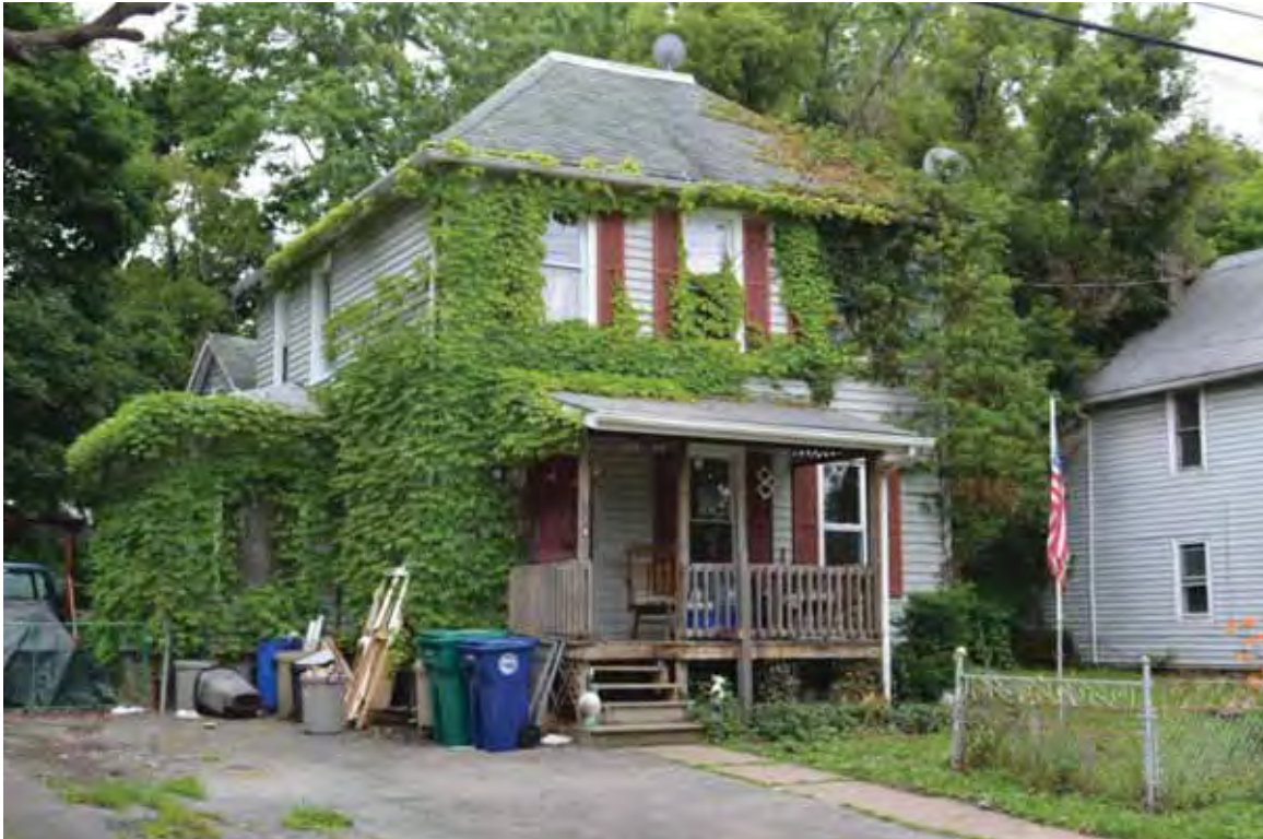
Photograph 4.188. 729 Willow Street, facing southwest (Panamerican 2014).
