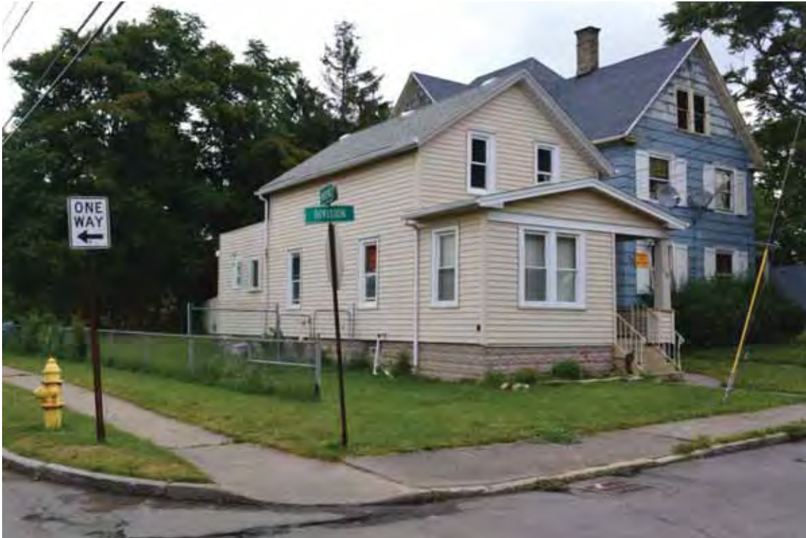
Photograph 4.69. 710 Division Avenue, facing northeast (Panamerican 2014).
