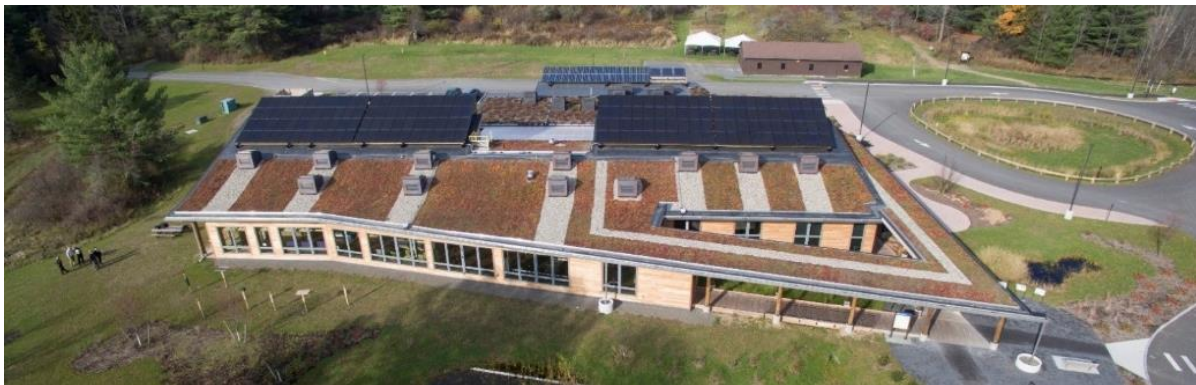
Dedicated in 2017, Five Rivers Visitor Center in Albany County is DEC's first Platinum LEED building, certified by the U.S. Green Building Council.
