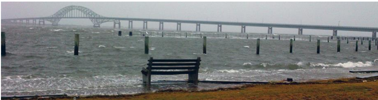
Empty pilings are visible at Robert Moses State Park on Long Island after Hurricane Sandy destroyed an extensive pier system (photo from October 29, 2012). The Fire Island Inlet bridge can be seen in the background.
