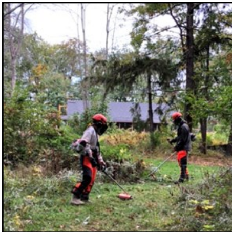
Maddie LeMere and Tad Townsend creating a defined path and edge to the newly installed Nature Center trail at Evangola State Park.
