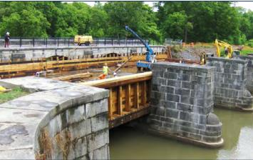
The aqueduct before (above left) and during its restoration (above right), showing the laminated timber trough being constructed within the limestone structure.
