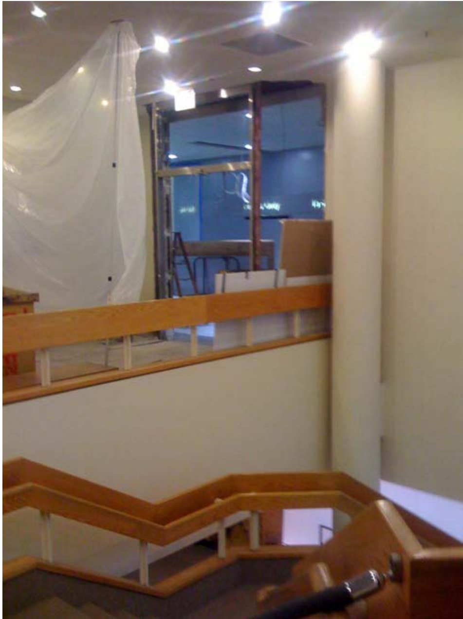
Figure 56: Construction photo during removal of door between the Narthex and the market building; source: St. Peter's Church Archive
