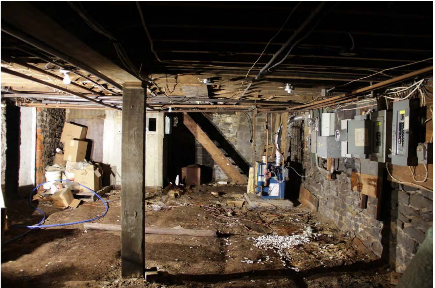
0015: View of basement.
