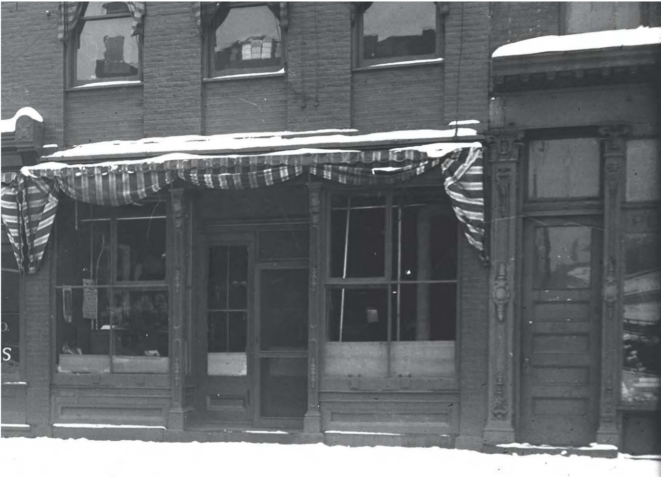
Closeup of Figure 7 showing detail of original storefront at 216 South Avenue.
