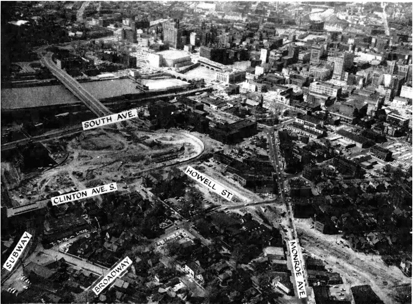
Figure 12B - Aerial view looking northwest over razing of neighborhood surrounding 216-222 South Avenue. "Father Rochester Can Point With Pride," Rochester Democrat and Chronicle (Rochester, NY), May 26, 1957.
