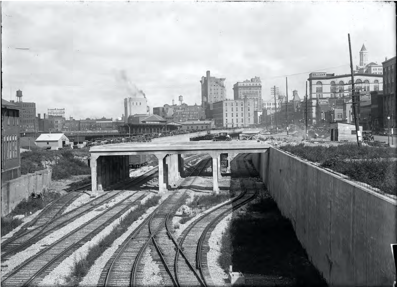
Figure 9 - 1926 view northward along new Rochester Subway in former Erie Canal bed, with 216-222 South Avenue far right. (Albert R. Stone Negative Collection, Rochester Museum and Science Center)
