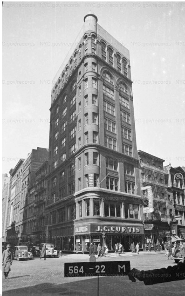
Figure 16: This circa 1940 Tax Department photo shows that the building's original cornice and storefronts had been removed by this point.
