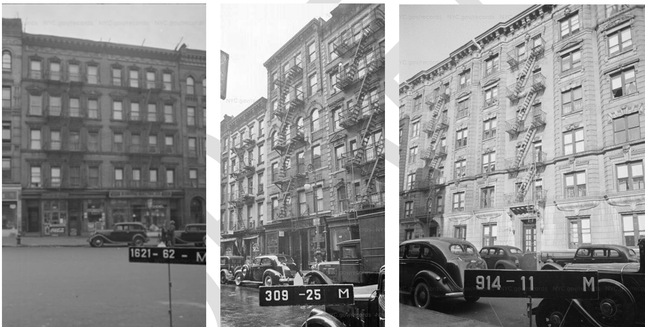
Figure 2: Tenements designed by Samuel Sass. From left to right: 18-20 E 116th Street (1897), 45 Ludlow Street (1898), and 211-229 East 33rd Street (1904). Photos from the 1940s NYC Tax Department photograph collection.
