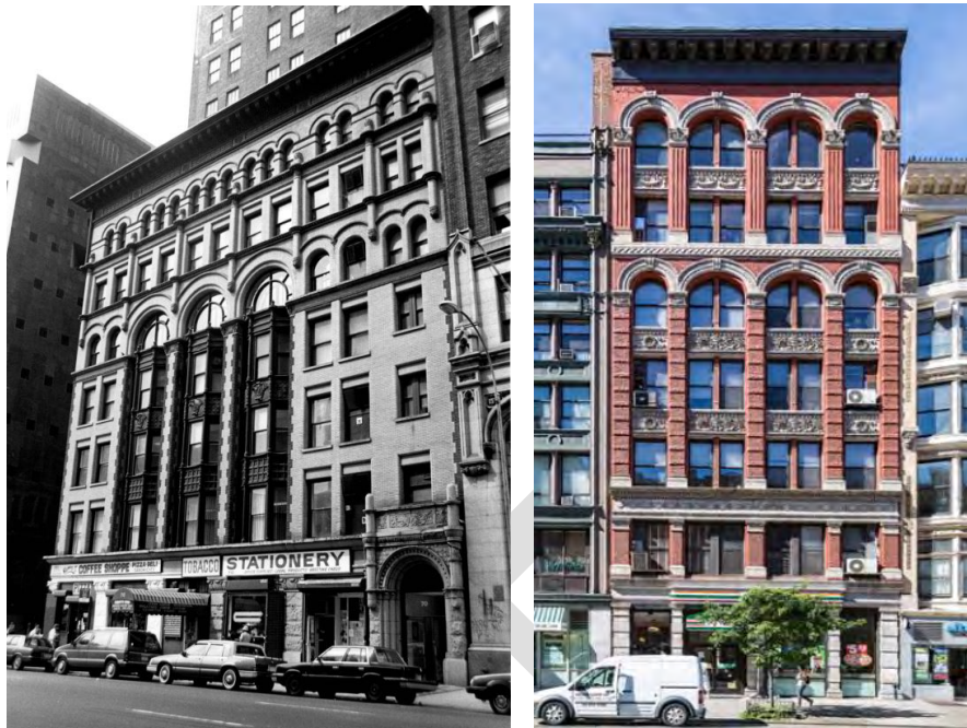
Figure 13: Left) The Ahrens Building at 70 Lafayette Street, designed by George H. Gribel and built in 1896 (Elisa Urbanelli), and Right) 244 West 23 rd Street, built in 1900 (newyorkitecture.com).
