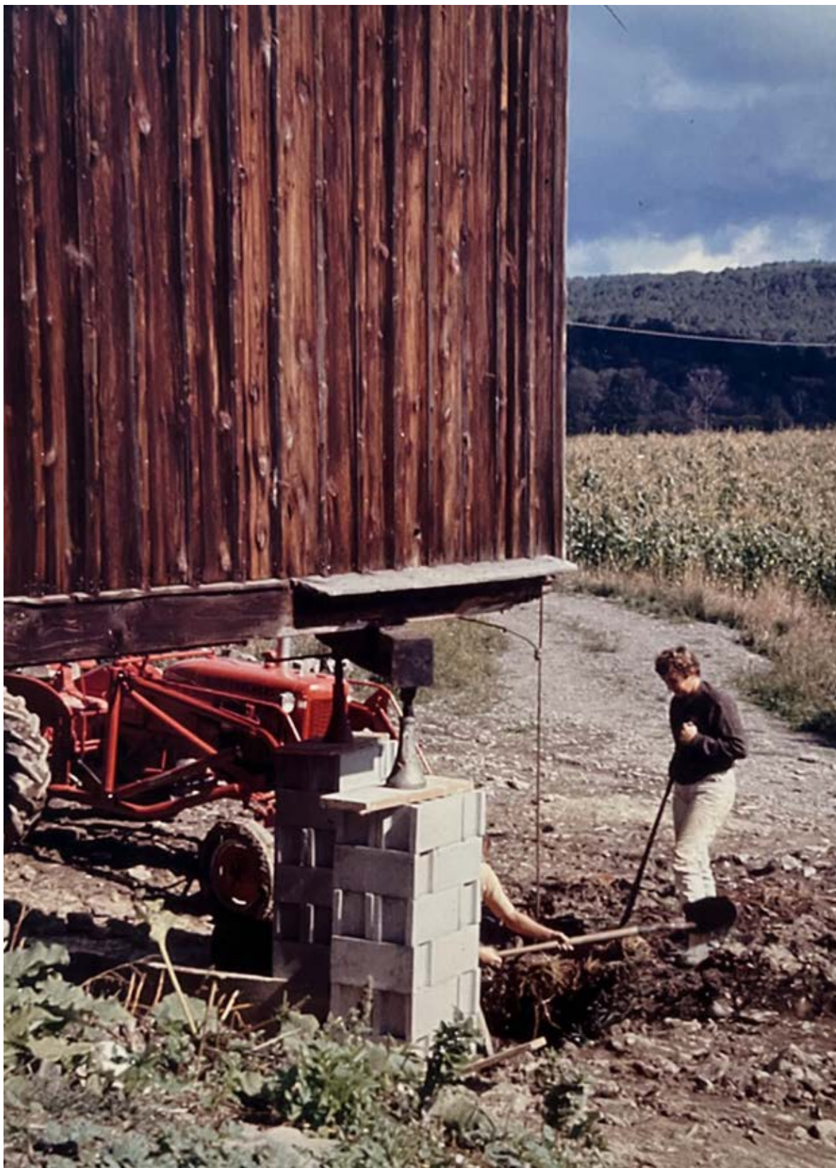
Figure 3: Vicky Romanoff and friend leveling barn and installing masonry block foundation.
