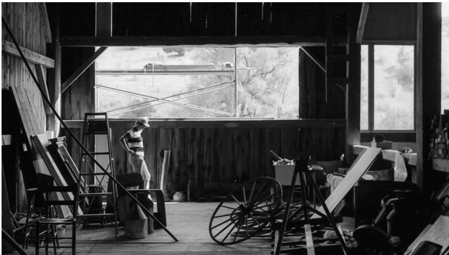
Figure 7: Romanoff working on the living room, with window opening cut but sash not yet installed.
