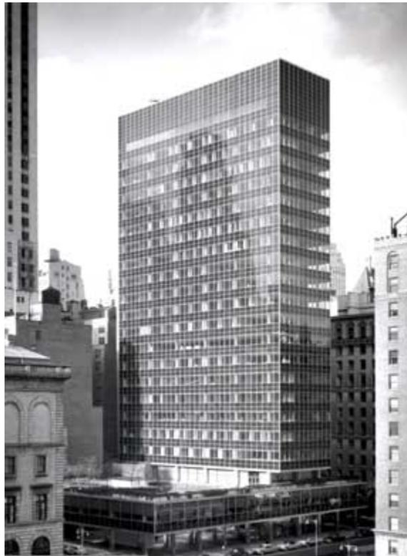
*Lever House in New York City: A landmark of a modern architecture. The failure of the original sealant materials at the glass curtain walls proved that not all modern replacement materials perform as promised, and sometime must be replaced themselves.*
