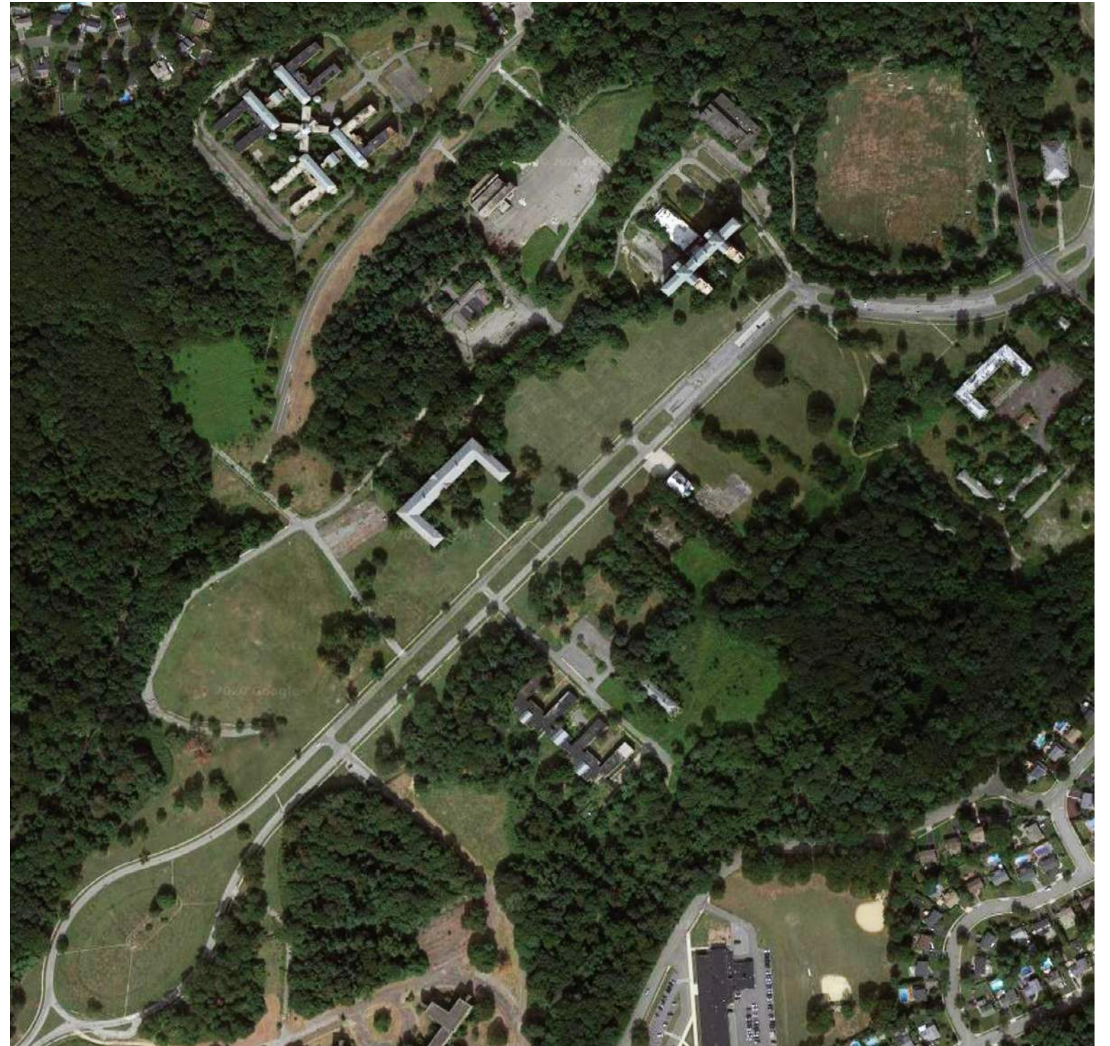
2020 AERIAL SHOWING EXTENT OF BUILDING DEMOLITION
