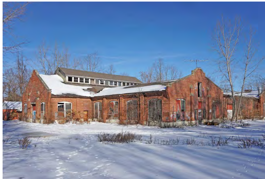
Old Laundry Building (Building 5)
