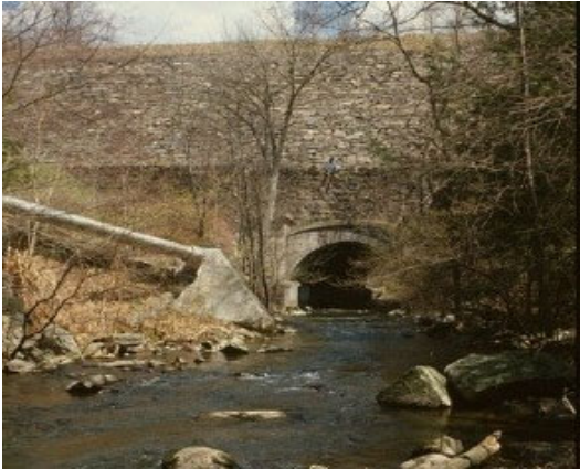
Mill River Culvert, Sleepy Hollow, Mile 9 Historic American Engineering Record
