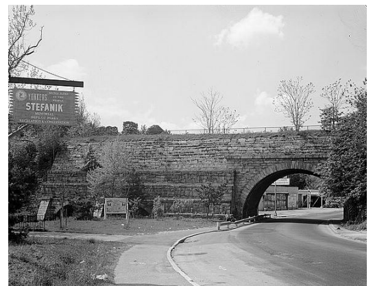
Arch Over Nepperhan Avenue Prior to Road Widening, Yonkers, Mile 22 Historic American Engineering Record
